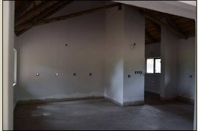
New kitchen, scullery and secure pantry area
