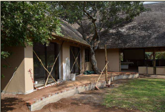
Preparing for paving to match the patio floor level so it is wheelchair friendly
