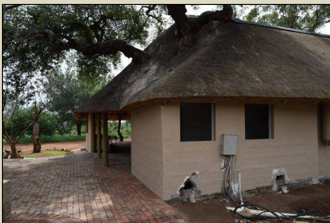
Access pathway replaced with paving
