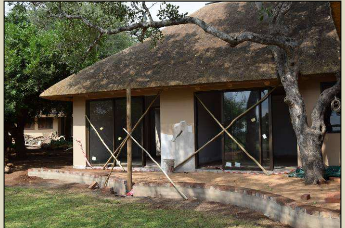
Preparing for paving to match the patio floor level so it is wheelchair friendly
