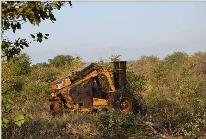
Specialised cutting machine in action on Buffelsbed
