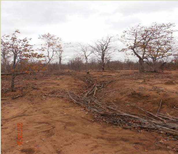
Branches packed into drainage lines/gullies
